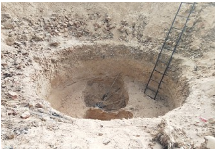
Underground hole for the 'cess pit'. The soil is very sandy and the sides of the hole started to fall in, so we had to start building quickly.
