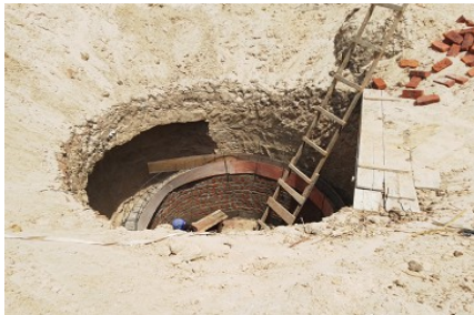
Underground hole for the 'cess pit'. The soil is very sandy and the sides of the hole started to fall in, so we had to start building quickly.
