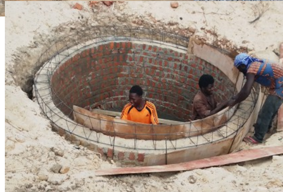
As you can see the bricks are placed sideways, rather than lengthways, with reinforced concrete rings, and the structure is circular. This is to make it strong enough to withstand the pressure of water.
