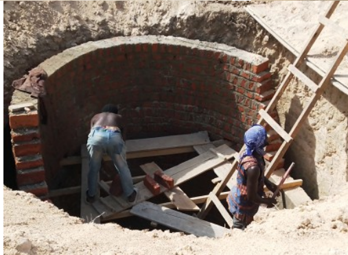
As you can see the bricks are placed sideways, rather than lengthways, with reinforced concrete rings, and the structure is circular. This is to make it strong enough to withstand the pressure of water.
