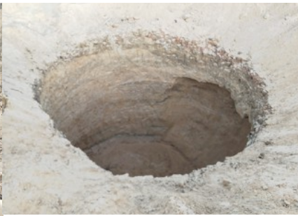
Underground hole for the 'cess pit'. The soil is very sandy and the sides of the hole started to fall in, so we had to start building quickly.
