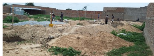
Digging foundation holes 3 metres deep
